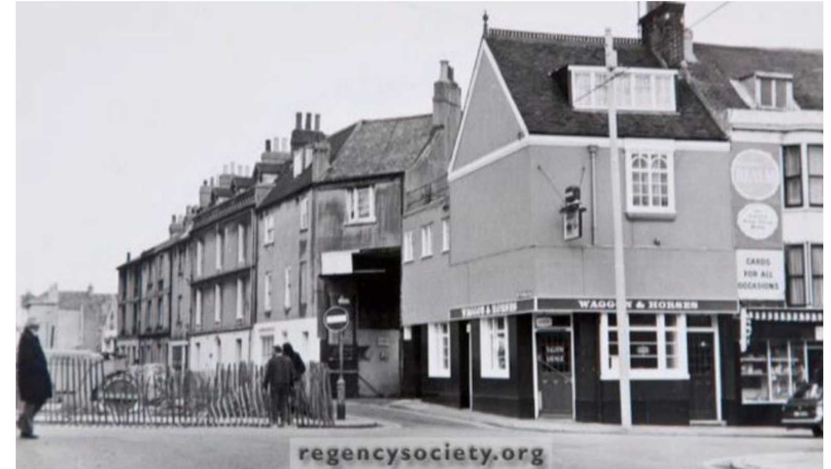
1972 - Jubilee street showing demolition
