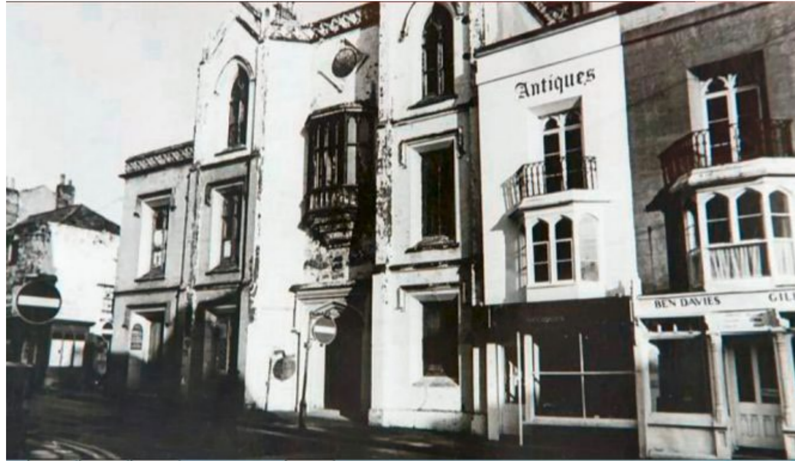
1971 - The national Central School and adjoining buildings
