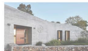
Tanawana Abbey Balduino Cortese Architects Board formed concrete
