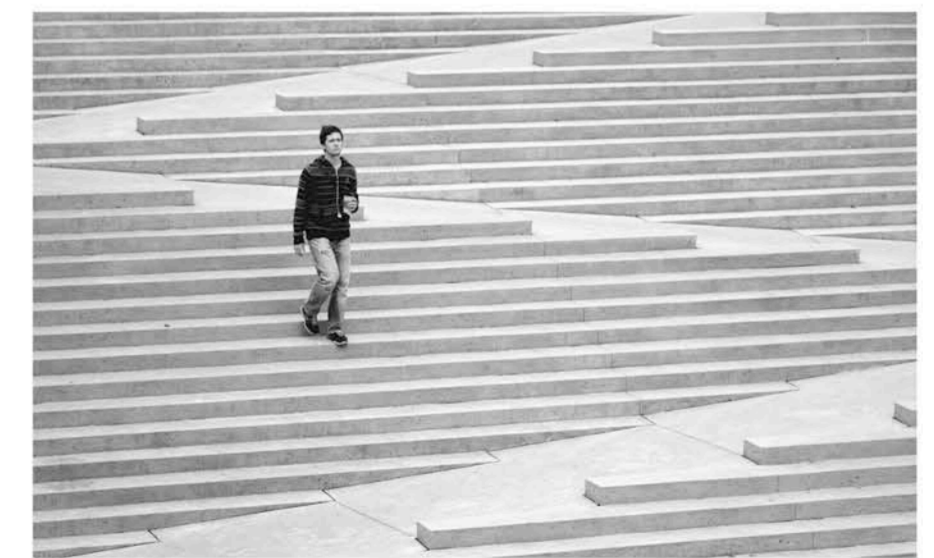
The "stomp" at Robson Square by Cornelia Oberlander, these stairs integrate a zig zag ramp to allow for maximum accessibility.
