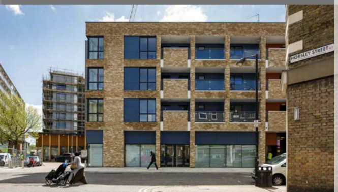
AYLESBURY ESTATE, LONDON Facade extends out to the path on the exterior of the dwellings
