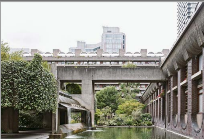
BARBICAN, LONDON Bridges which intertwine to create a labyrinth of paths through site without being directly next to a unit on the upper levels
