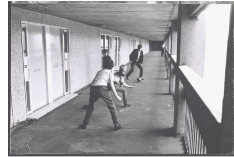
Park Hill Housing Estate
