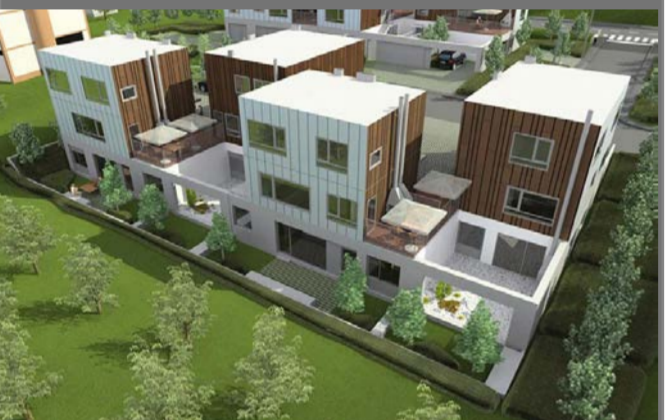
RURAL MAT njiric + arhitekti Small outdoor spaces privatised from the language and organisation of the buildings
