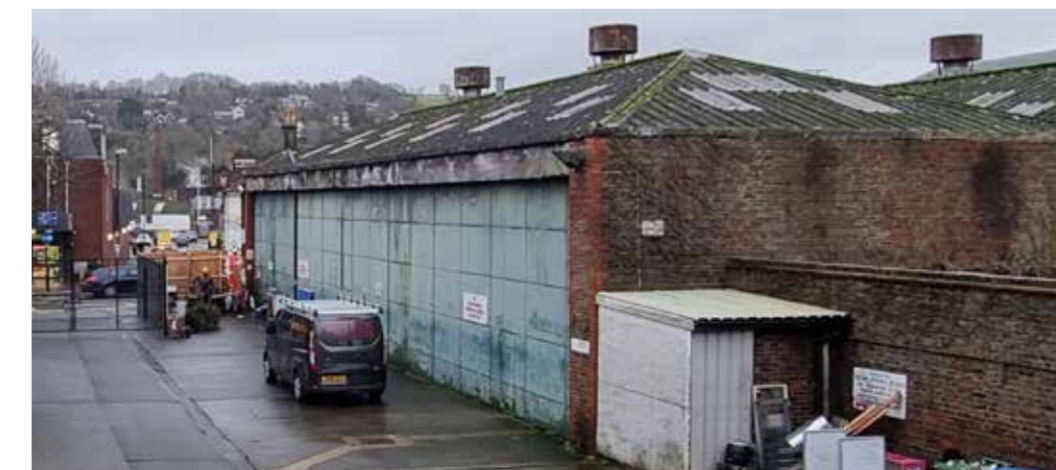
Front view of building
