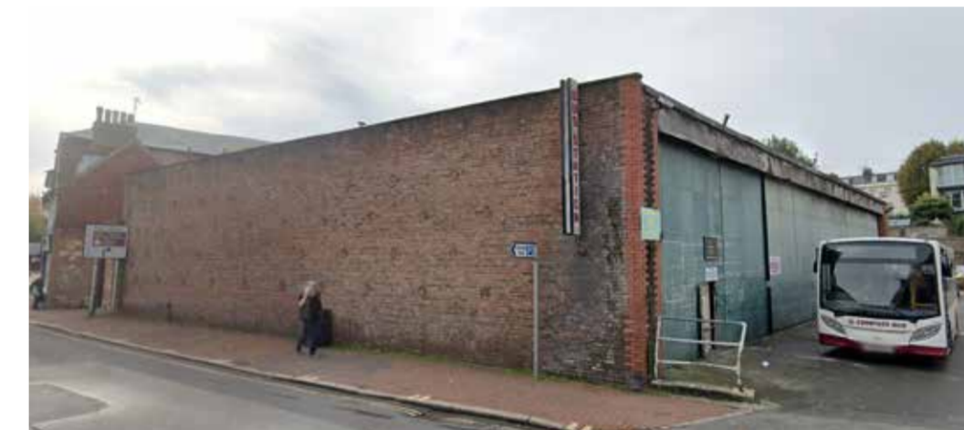
Exterior view of building
