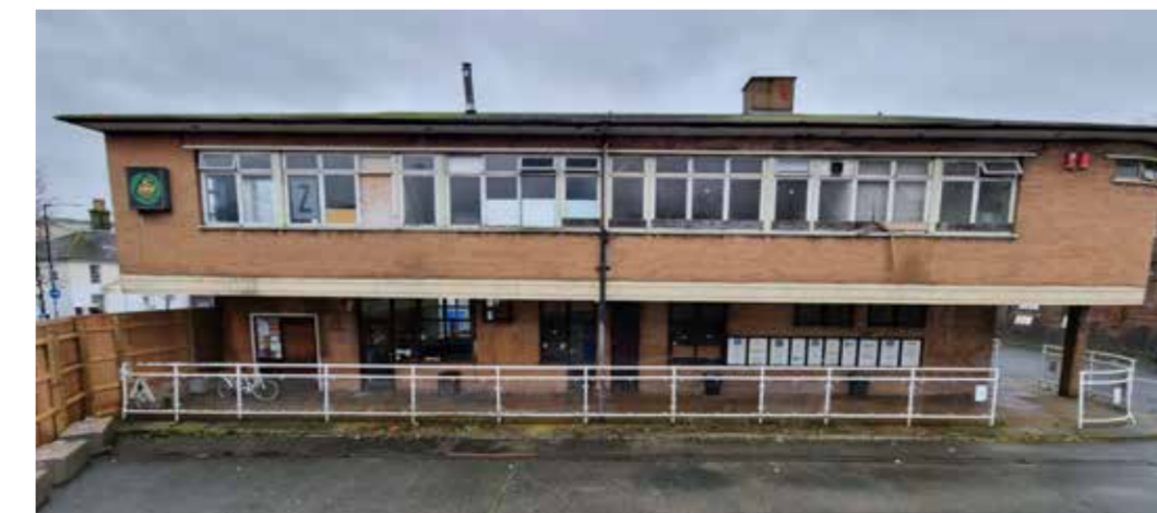
Side view of building
