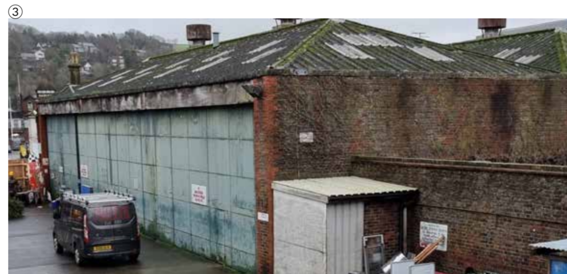
Space between the two buildings
