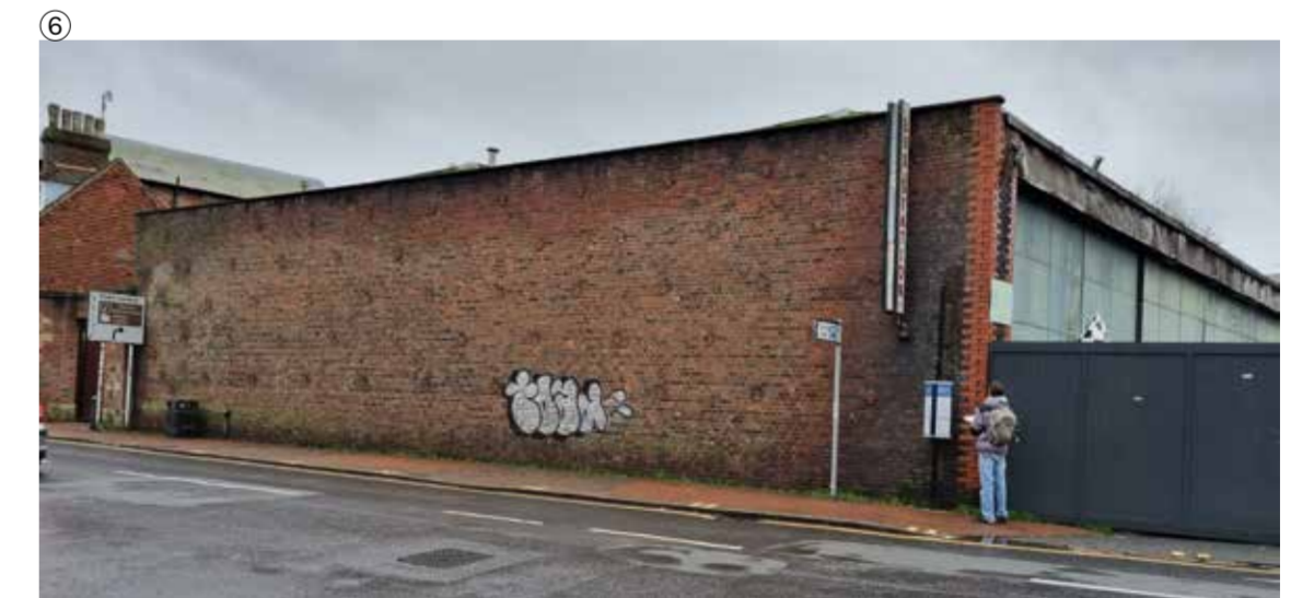
Side view of the Bus Depot
