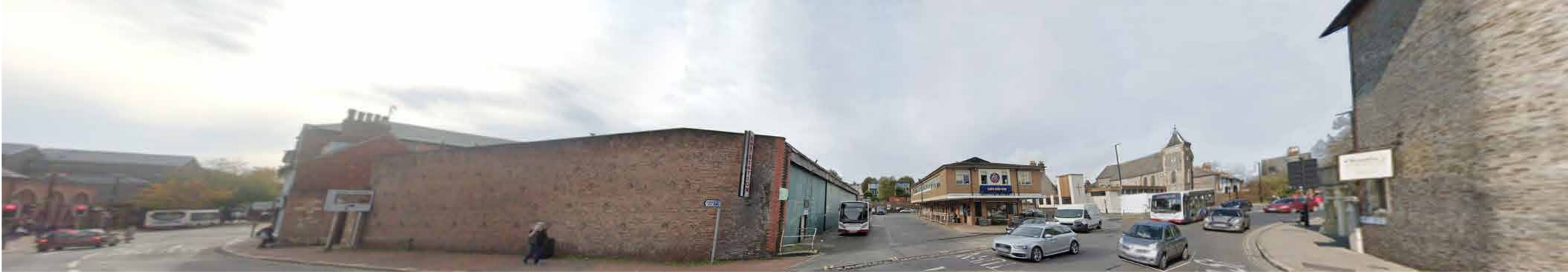
Site from Street View cr: Google
