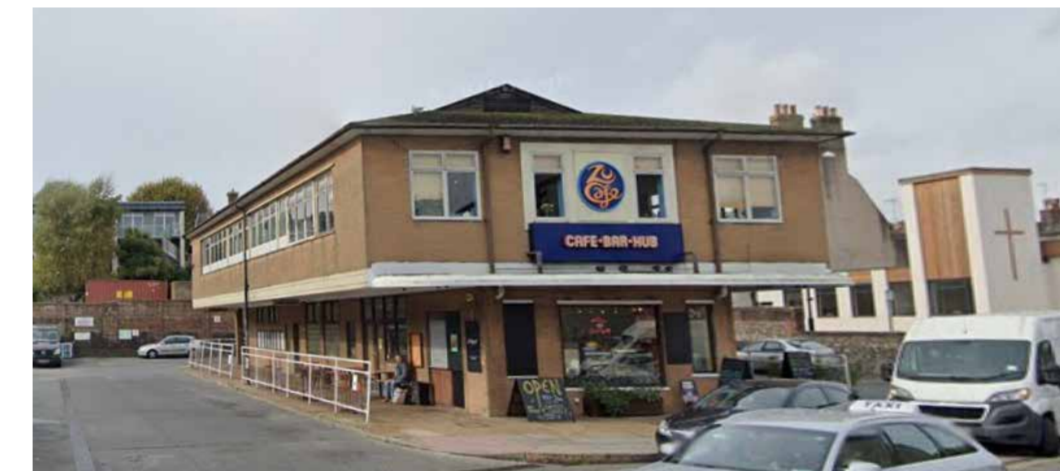
Front view of building
