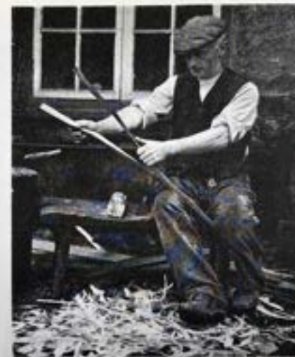
86. Completing the clearing by hand.
