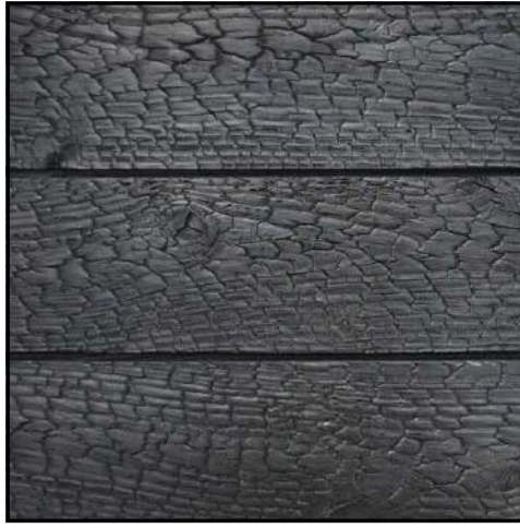
Image of Burnt Ash Closeup
