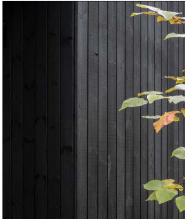
Image of Burnt Ash Cladding
