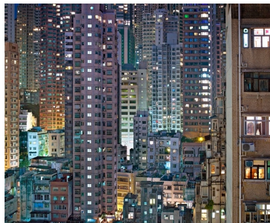
Fig 28. Hong Kong's Dense Tower Blocks
