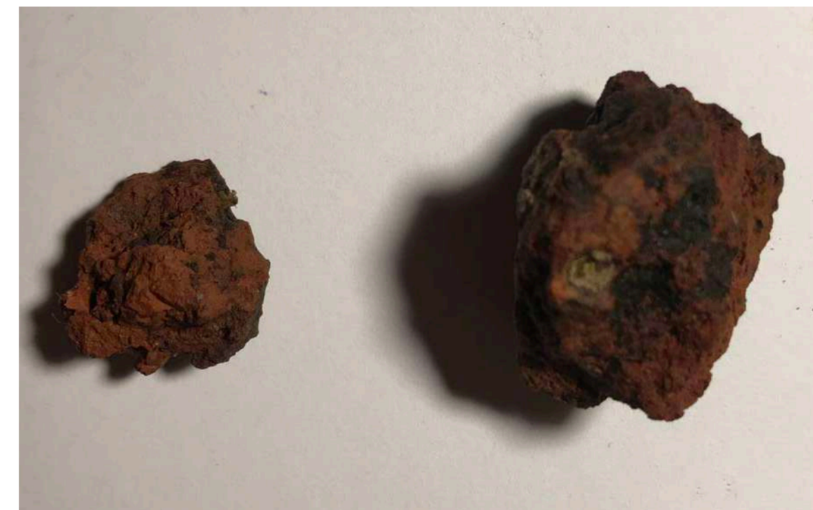
Crumbled brick from West Hill House facade
