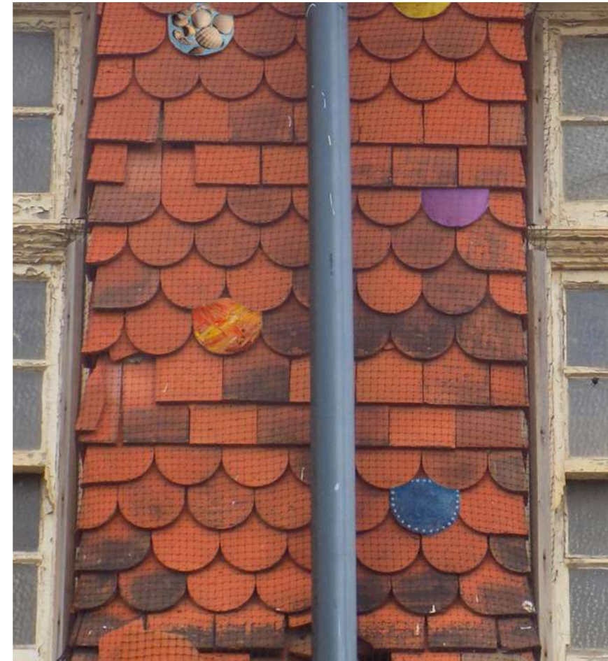
Repairing With Colourful Tiles
