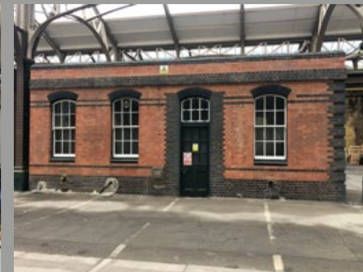
Ex platform waiting rooms
