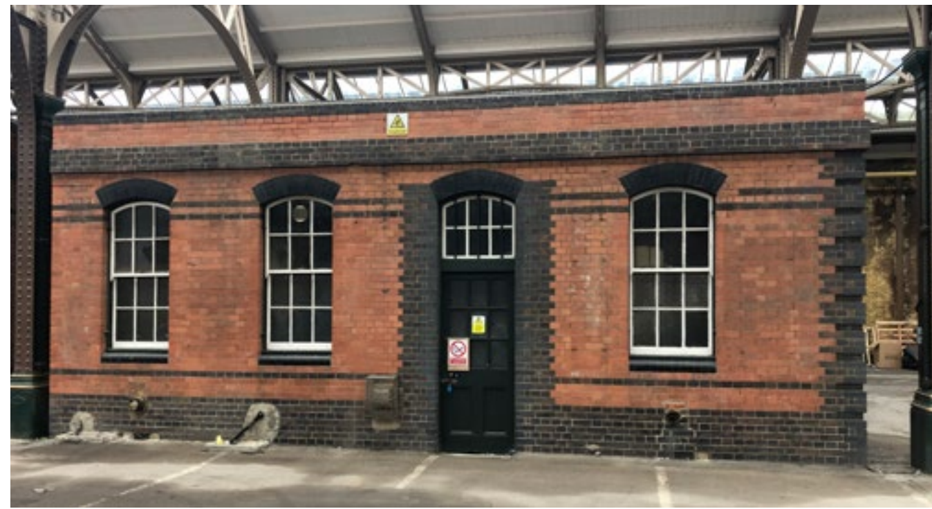
Waiting room at western end of the station
