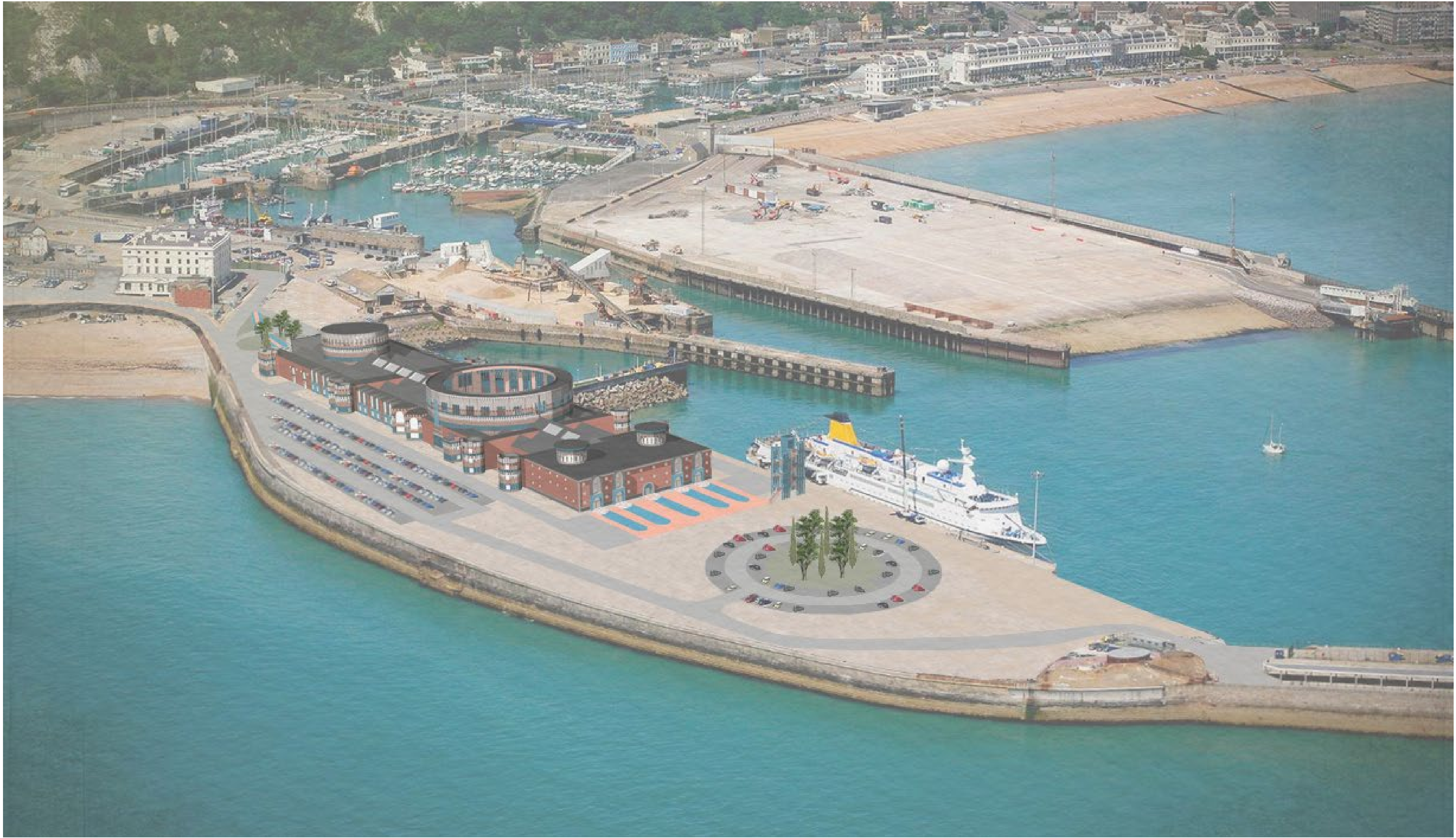
View looking north up the western dock
