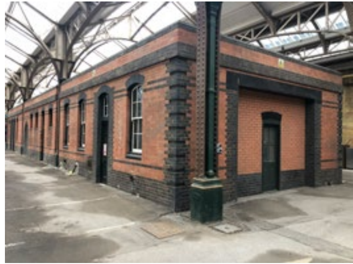
Red & black bricks on site
