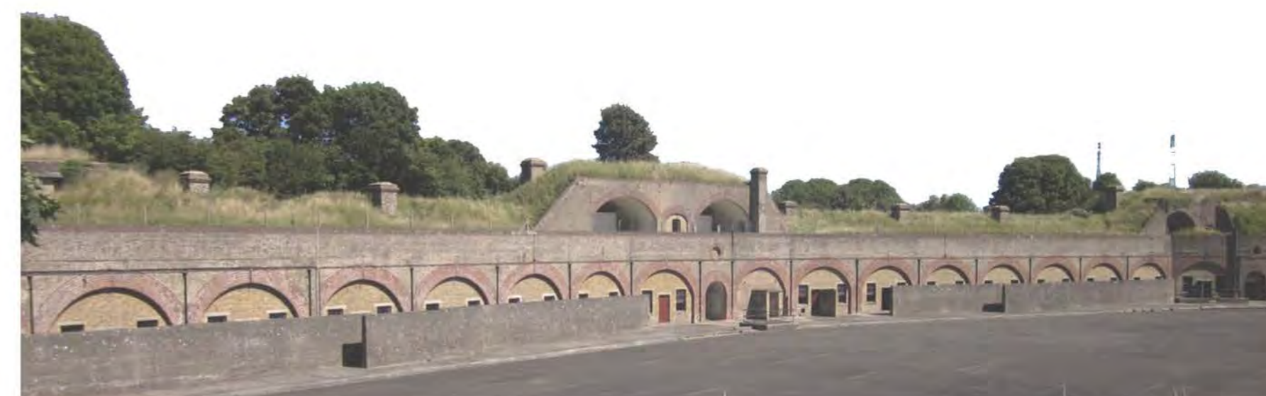
South elevation of Fort Burgoyne
