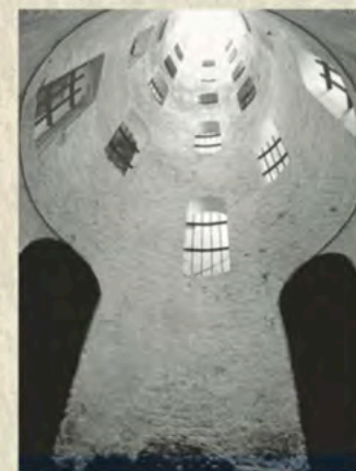
The Grand shaft a 140ft triple staircase, that linked the town to the forts.
