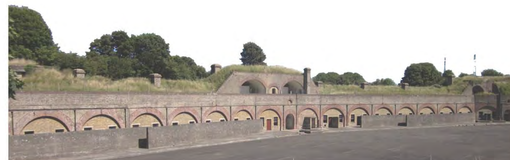
South elevation of Fort Burgoyne
