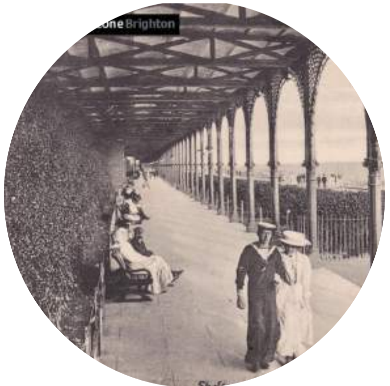
Madeira Drive - terraces and an accessible walkway that included a smoking room, café, a skating ring, and a music conservatory. (Live music performances occurring regularly for all classes) GREEN, B. H. B. 2017. The story of 'Maddy' - Brighton's historic Madeira Drive [Online]. Available: https://building-green.org.uk/2017/04/18/the-story-of-maddy-brightons-historic-madeira-drive/ [Accessed December 2021].
