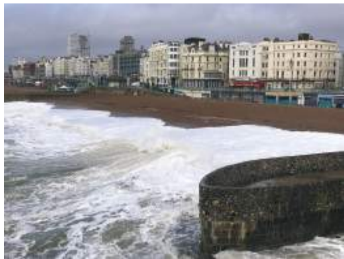
Landing stage beside the pier providing side views of the pier structure.
