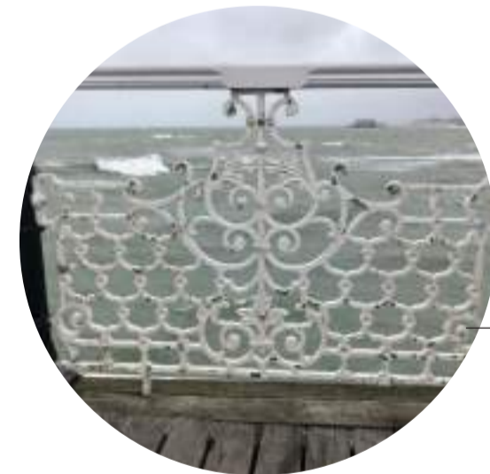
Organic ornamental cast iron fences along the whole promenade.
