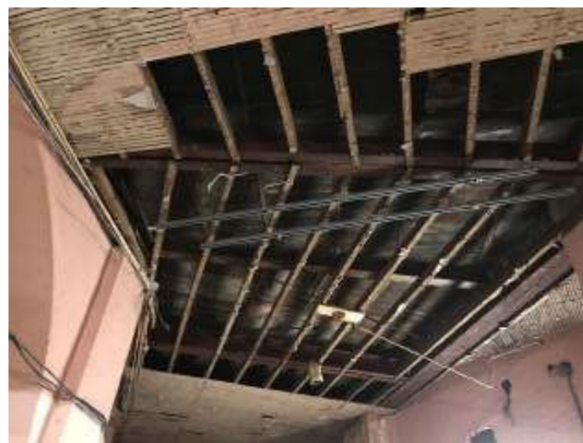
ceiling restoration in process
