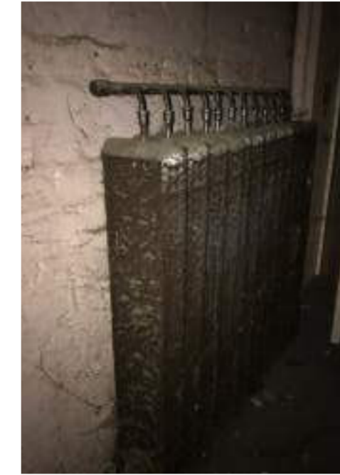
historic radiator to preserve
