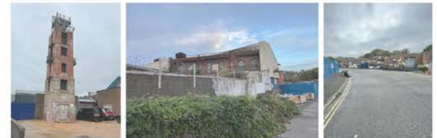
Lewes Fire Station
