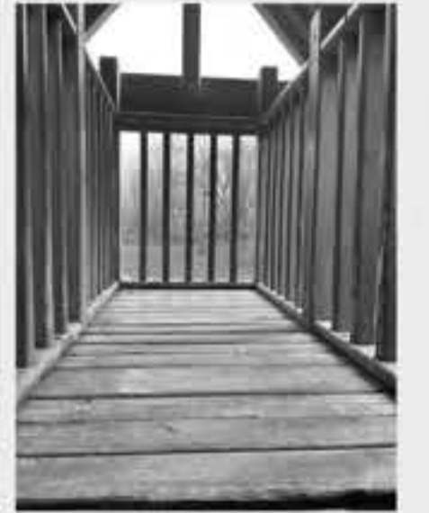
Pillars for walkways
