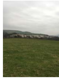
Railway and quarry
