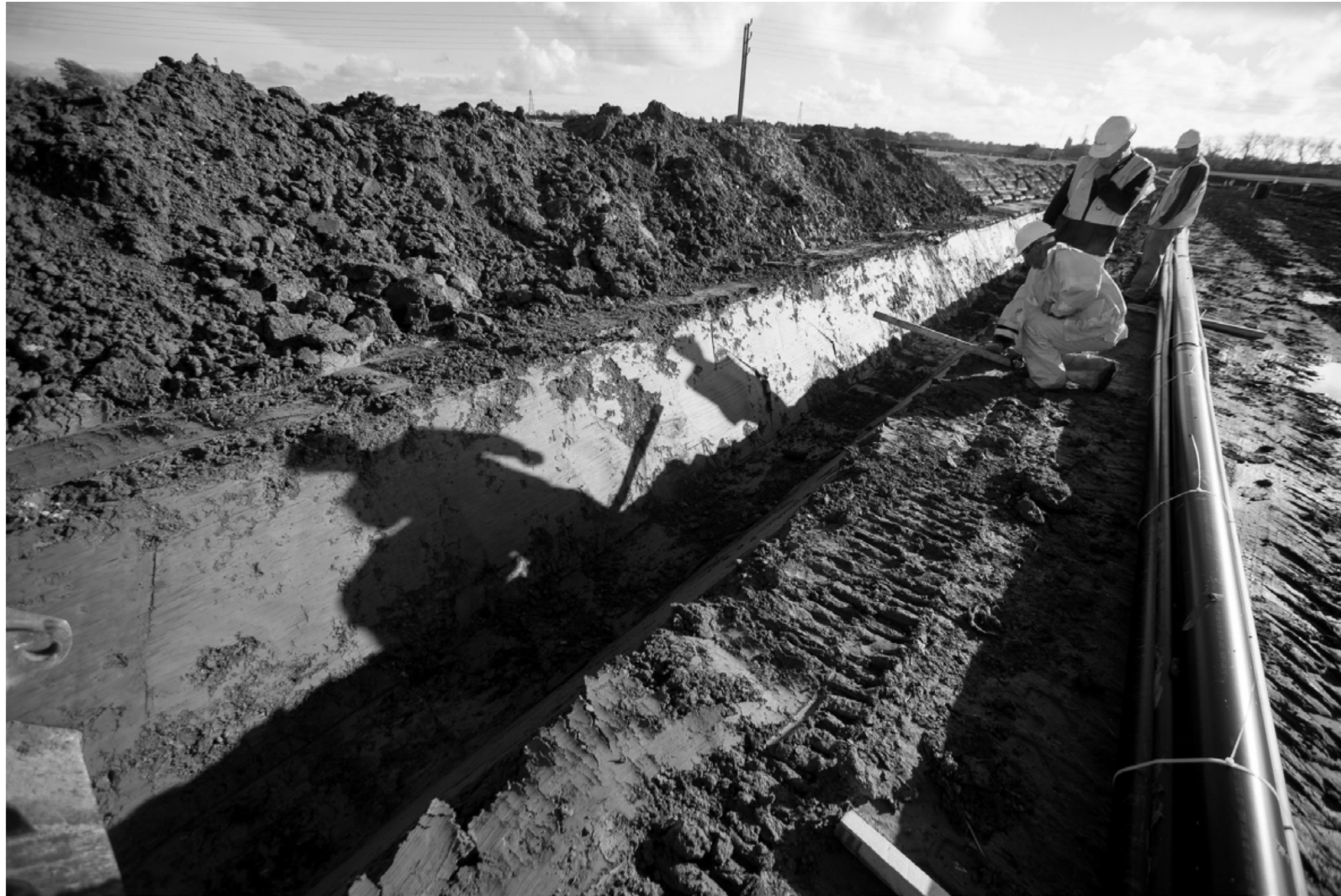
Workers inspecting the Rampion onshore cable trench
