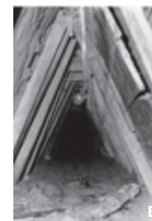
• Tunnel 29 Joachim Rudolph, 1961, Under The Berlin Wall. https://www.express.co.uk/news/world/1202179/Berlin-wall-anniversary-bbc-podcast-tunnel-29
