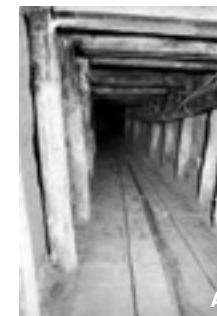
• Tunnel 29, Joachim Rudolph, 1961, Under The Berlin Wall. https://www.express.co.uk/news/world/1202179/Berlin-wall-anniversary-bbc-podcast-tunnel-29
